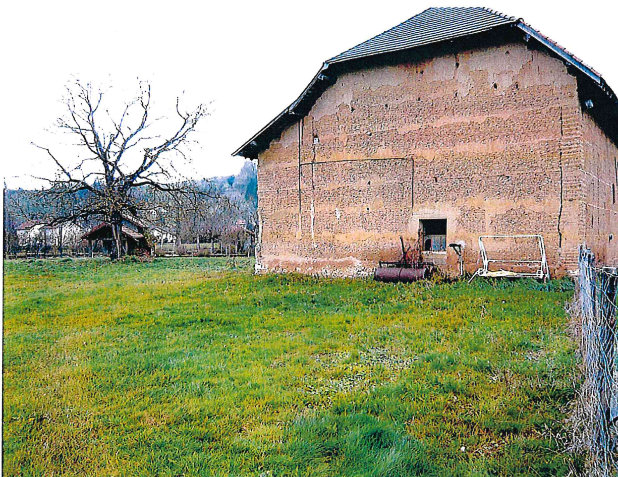
FIGURE 6 : GRANGE A REHABILITER
